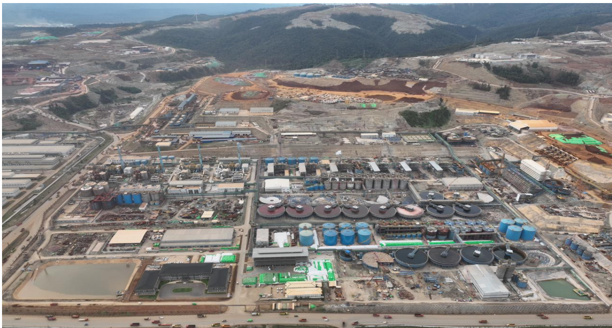
PT BSE HPAL aerial view
