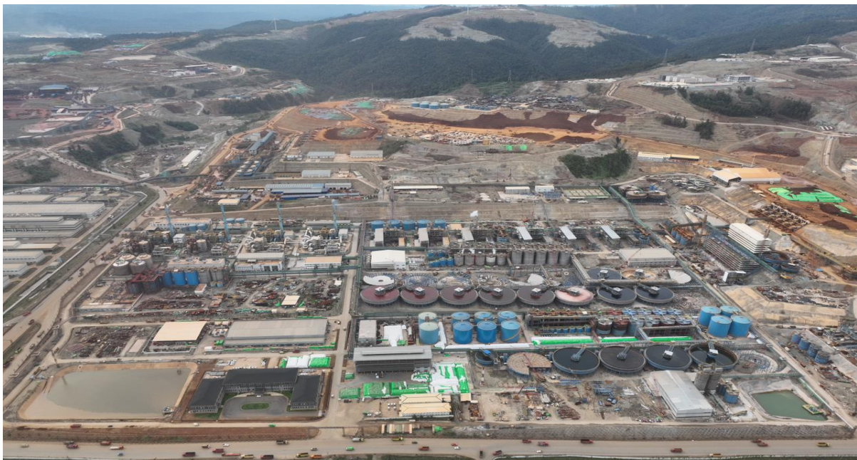
PT BSE HPAL aerial view
